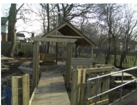
KS2 outdoor classroom is nearly complete
